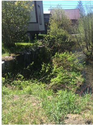
Location where Kingsbury Branch crosses under Church St.
