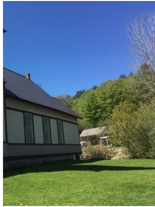
A subsurface infiltration chamber system is proposed along the road in the lawn north of the church.
