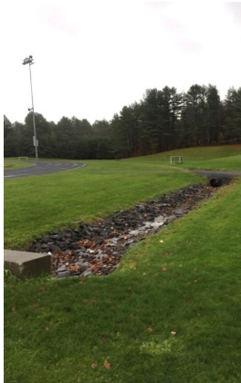
Stormwater from the school is directed to a series of swales south of the track. Drainage from the swales flows to a low point beyond the tree line.
