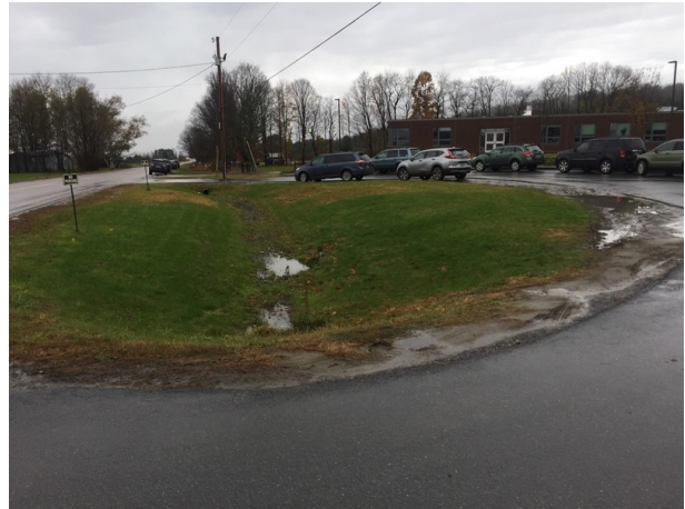
Figure B13. Stormwater draining to the pictured greenspace will be treated in a bioretention.
