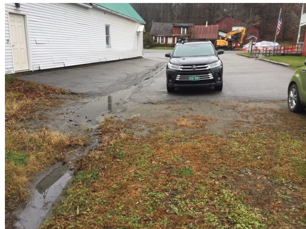
Figure C13. A subsurface chamber system is proposed to treat runoff from the Fire Station and Post Office site.
