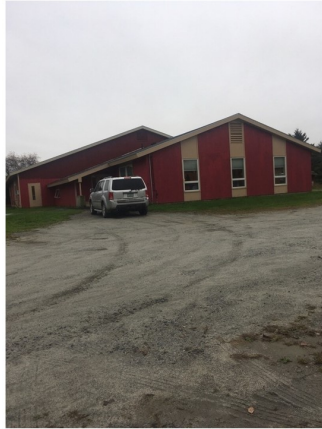
Stormwater from the western half of the Calais Elementary School site flows over the gravel parking lot to a ditch running parallel to the cow pasture. The ditch eventually drains to a wetland south of the school.
