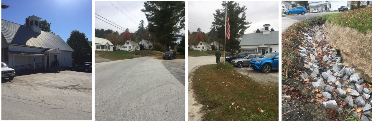
Stormwater from the Post Office runs over the pavement into a culvert, down a ditch along Moscow Woods Rd and into the Kingsbury Branch.
