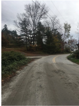
Drainage from Moscow Woods Rd is causing erosion in the same gully that receives drainage from Batten Rd by the Post Office (pictured).
