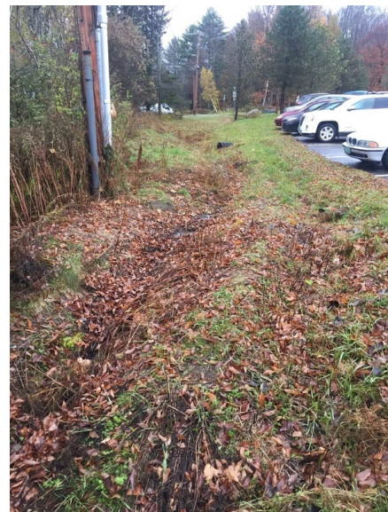
Figure B10. Stormwater draining from the pictured swale will be treated in a gravel wetland.
