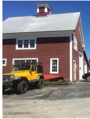
A new catchbasin and pipe connection at the garage will direct stormwater to the new subsurface system.
