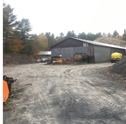
Figure A12. An infiltration basin is proposed for the Calais Town Garage site.
