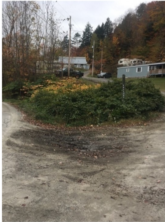
Proposed location for an infiltration basin. Stormwater collects in this area and is piped across the street to an eroding gully.
