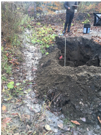
Figure A28. An excavator was used to assess soil conditions and infiltration potential.
