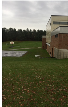
Drainage from the building, parking lot, and athletic fields is directed to the swales.
