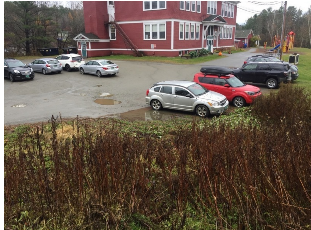
Figure C9. Stormwater runoff from the Woodbury School’s parking lot will be treated in a gravel wetland.
