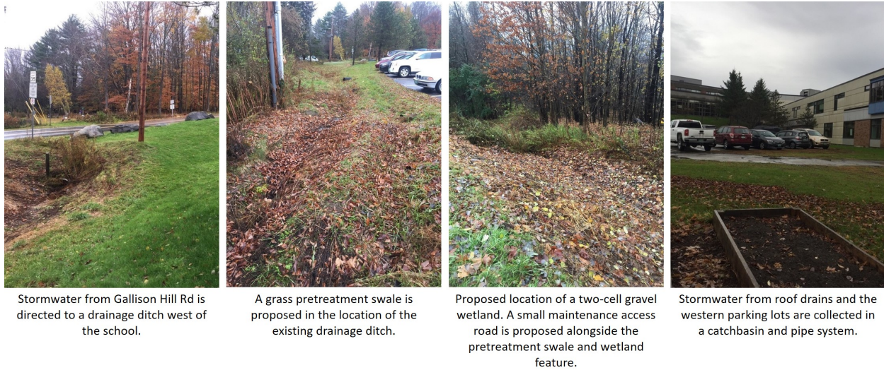
Figure B17. The proposed retrofits are described in the above photos.
