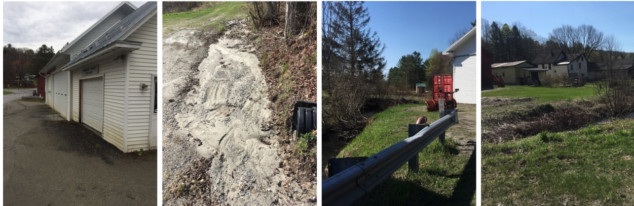
The Women’s Auxiliary Fire Department and Woodbury’s Food Shelf share a building on Valley Lake Rd. Gutters from the roof will be directed to a proposed dry well located behind the building.
